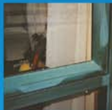
Examples of solvent misuse on a powder coated surface after a 3 year period.
